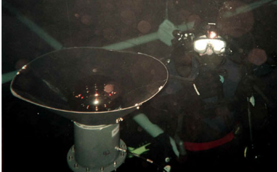
Figure 5.5: A diver working on a PMT during a repair operation. The baffle and the PMT encapsulation can be seen.
