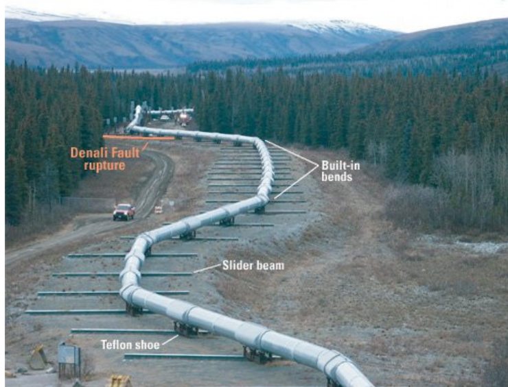
Trans-Alaska oil pipeline. Notice the damage.
