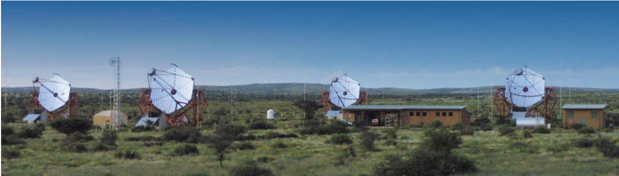
Fig. 1 The H.E.S.S. telescope array [1] in the Khomas Highland of Namibia at an elevation of 1800 m a.s.l. The four 13 m telescopes stand at the corners of a square with a side length of 120 m.
