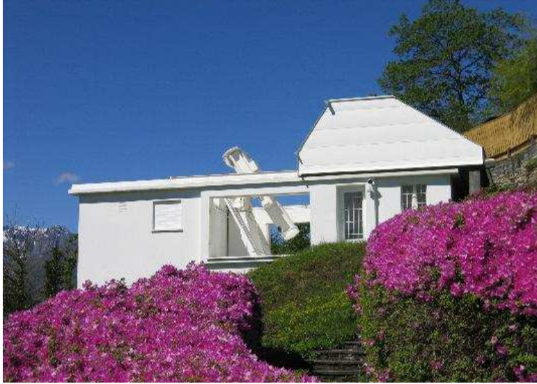
Fig. 1. IRSOL Observatory. In the left part of the building there is the observing room, while the spectrograph room is underground. All is painted white with titanium dioxide. The institute is located 500 m above sea-level, above the city of Locarno, Switzerland.
