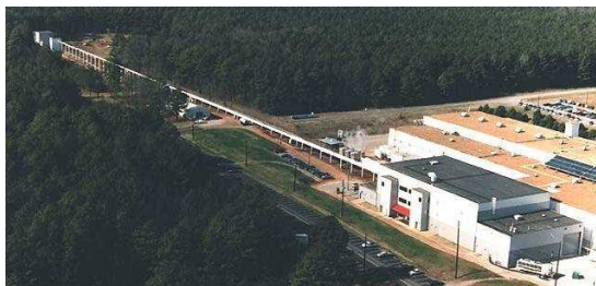
Fig. 5. The XRCF at MSFC. The building to the left houses the X-ray sources, filters, and monochrometers. In the building on the right is the large thermal vacuum chamber, at a distance of 525 m from the source building. The chamber accommodates the Chandra 10-m focal length and full illumination of the 1.2 meter diameter optics.
