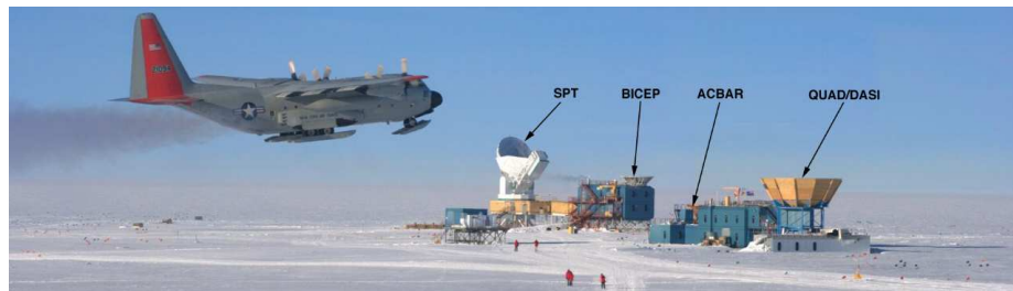
Fig. 2 The Martin A Pomerantz Observatory (MAPO) in the “Dark Sector” of the US Amundsen-Scott South Pole Station. From left to right, the telescopes are the 10 m South Pole Telescope (SPT), the 25 cm BICEP, the 2.1 m Viper with ACBAR and the Degree Angular Scale Interferometer (DASI) with QUaD. §4.2 provides further information on their capabilities. A ski-equipped LC130 aircraft, as used for supplying the station with all personnel and cargo, takes off from the ski-way to left. Several humans seen to foreground provide a sense of scale. They are traversing across the ski-way from the main South Pole Station base 1 km away (behind the camera). Image courtesy of Steffan Richter.
