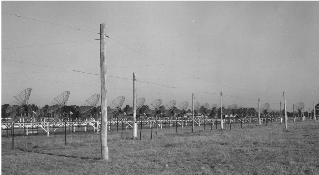
Figure 39 - Suspended dipoles of the Shain Cross at the Fleurs field station. In the background are the aerials of the Chris Cross.
