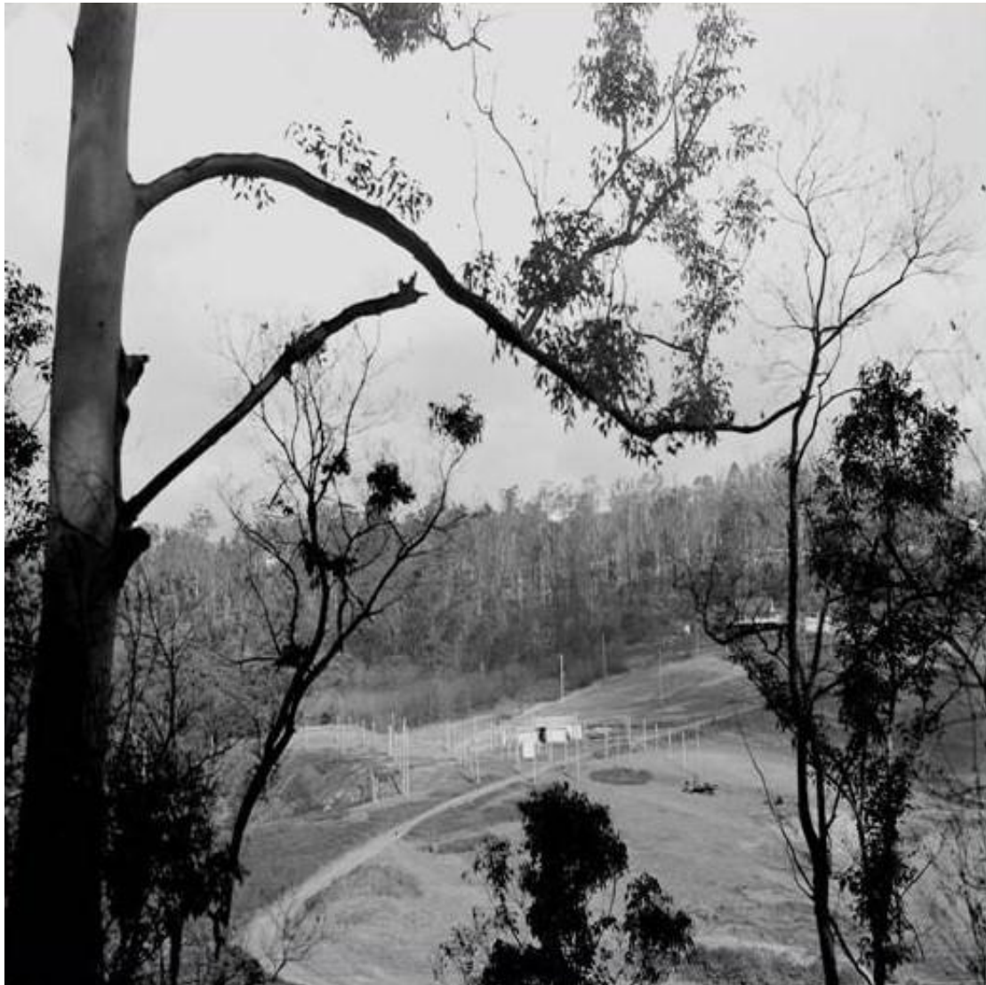
Figure 28 - The Hornsby Valley field station in July 1952 showing the 18.3 MHz eight half-wave dipoles connected in phase and raised 0.2 wavelengths above the ground.
