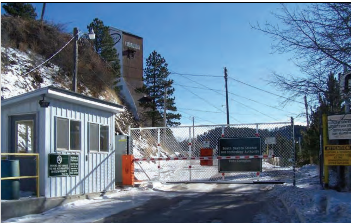
Figure 5.5.2-4 Ross Complex entrance gate.
