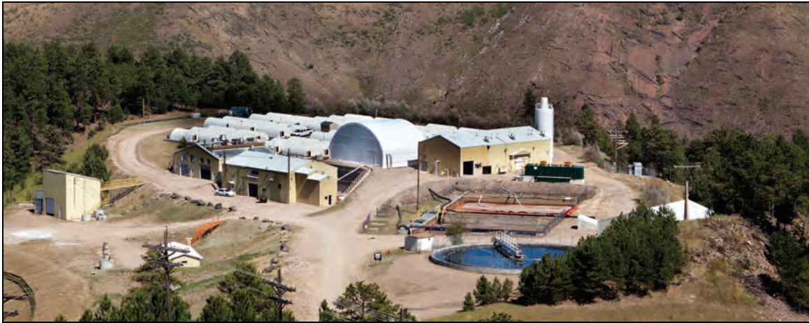
Figure 5.2.6.4.1-1 Waste Water Treatment Plant. [John Scheetz, DUSEL]
