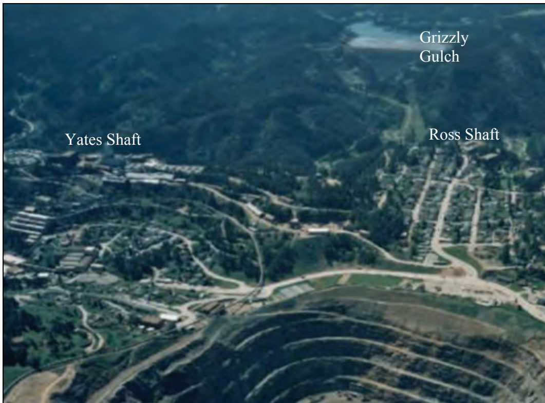
Figure 5.4.3.12.1-1 Aerial view of Open Cut workings looking to the south.
