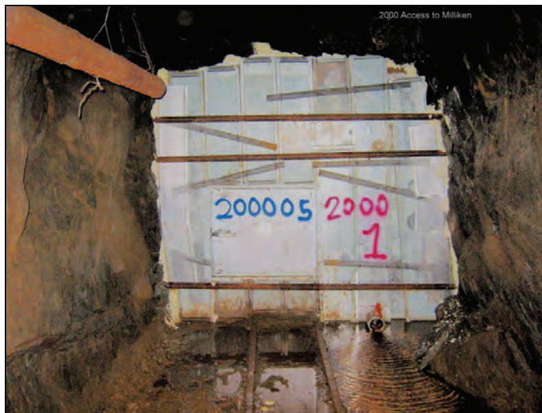
Figure 5.4.3.8.1-2 Kennedy Stopping on the 2000L. [SDSTA]
