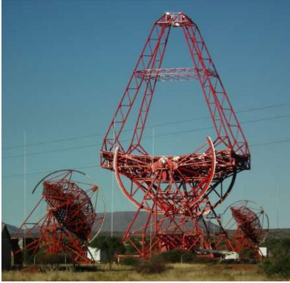
Figure 15: The steel structure for the 600 m<sup>2</sup> H.E.S.S. II telescope. Mirrors and camera will be installed in the first half of 2012. (Note that the H.E.S.S. II telescope is located in between the two H.E.S.S. I telescopes shown in the image, not in the foreground). Figure courtesy of the H.E.S.S. collaboration <http://www.mpi-hd.mpg.de/hfm/HESS/>
