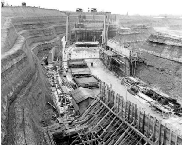
Fig.12: The excavation of the ISR tunnel
