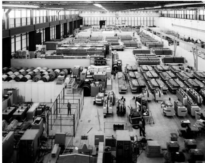
Fig. 15: Assembly, testing and storage of ISR magnets in the West Hall
