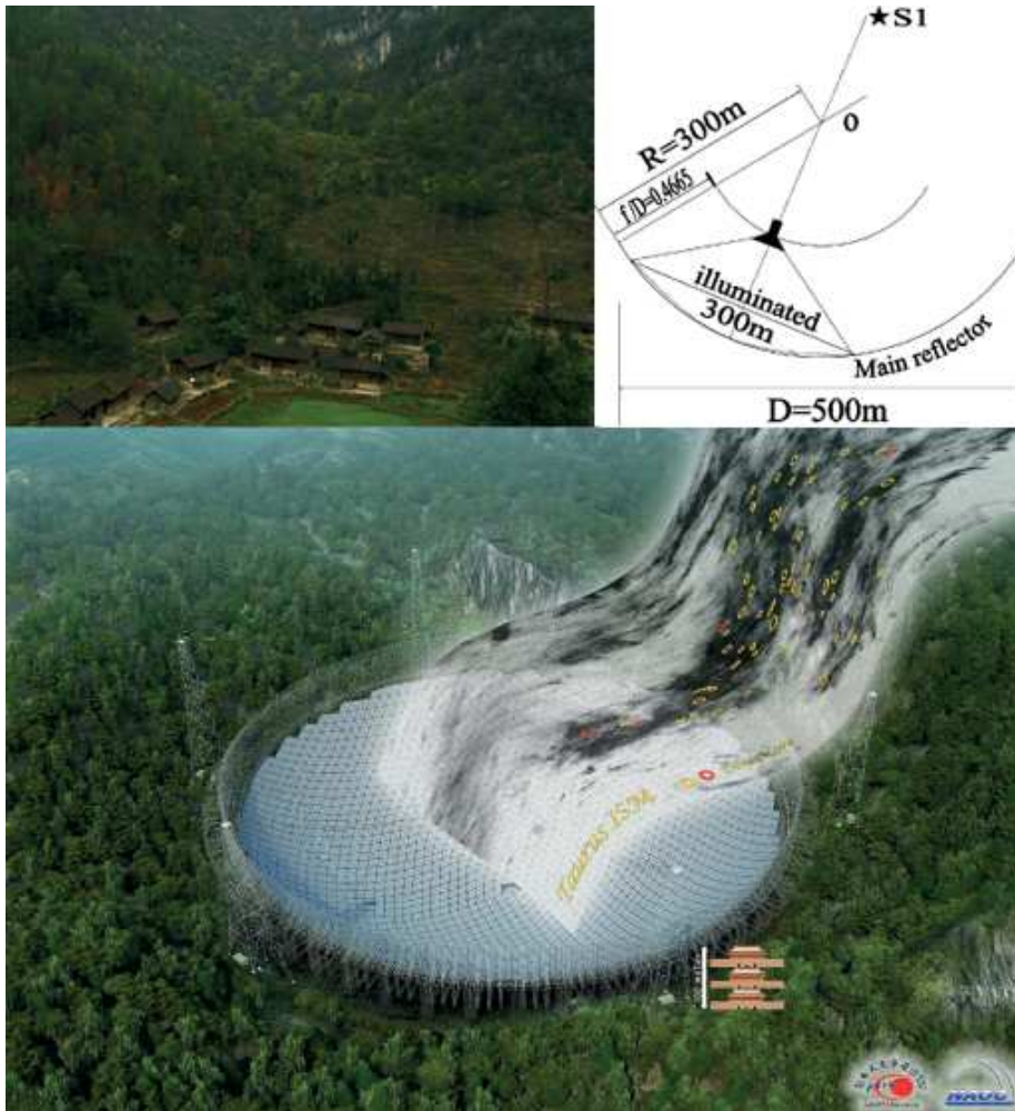
Figure 1. Upper Left: Partial view of the original site as seen in Nov of 2009. Upper Right: FAST optical geometry. Lower: A 3D model of FAST.
