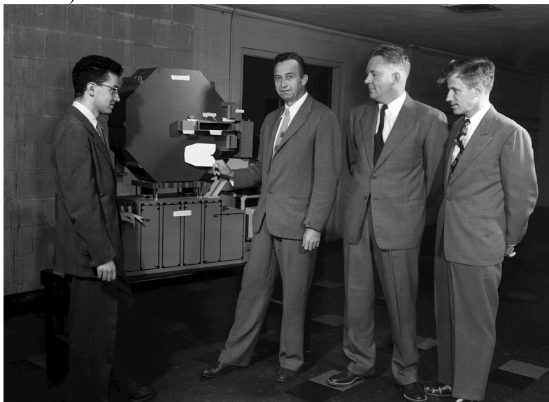
Figure 5. Courant, Livingston, Snyder and Blewett next to model of Cosmotron C-shaped magnet. Livingston holds cutout of magnet for strong focusing machine of same energy.
