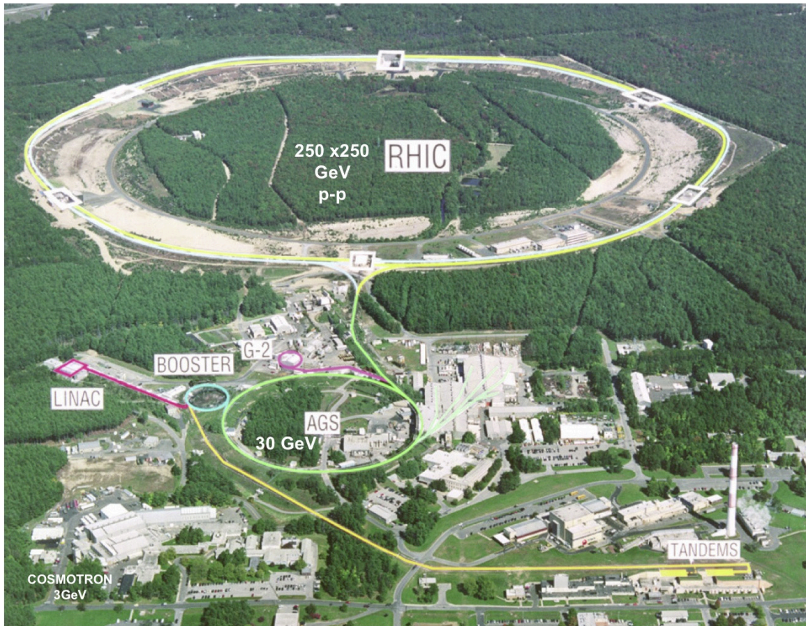
Figure 3. A closer view of RHIC at Brookhaven National Laboratory. The large circle without tree cover is excavation related to the enclosure of the RHIC machine. The labeled lines show the Linac, Booster accelerator for polarized proton injection, the tandem van de graaf accelerator and transfer line to the booster, and the AGS which accelerates the beams to an energy of 22 GeV per nucleon \times Z/A where Z and A are the atomic number and weight of the nucleus.
