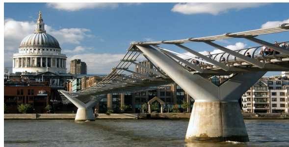
Figure 9: The London Millennium Bridge.
