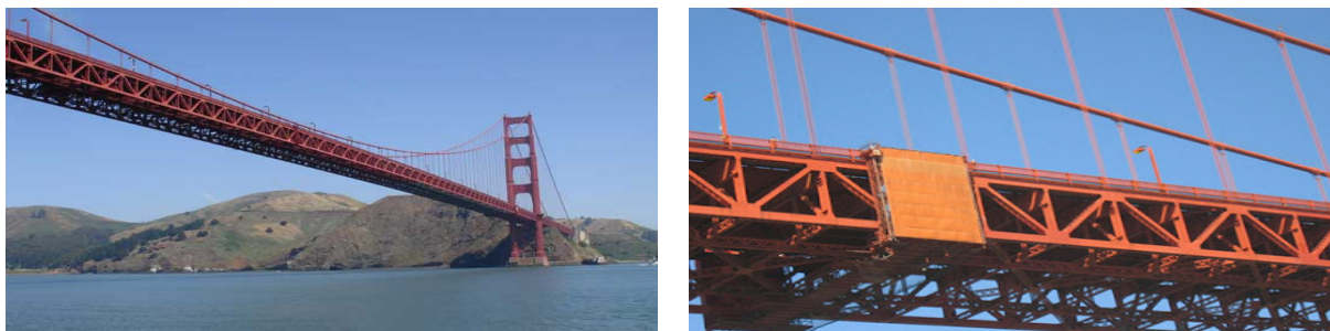
Figure 4: Girder at the Golden Gate Bridge.
