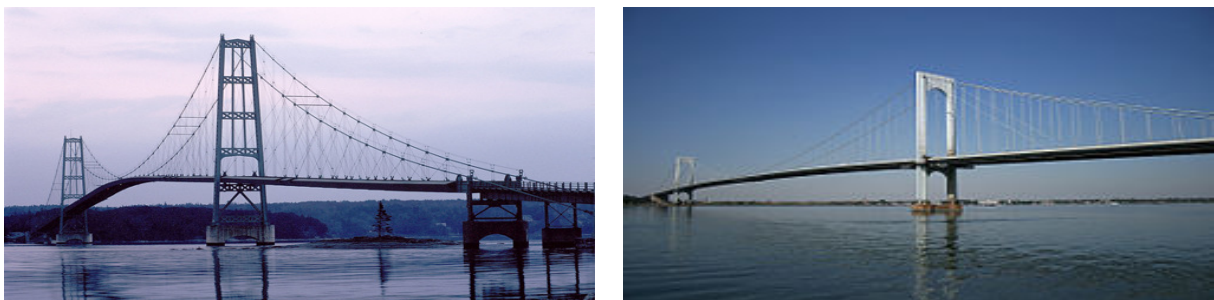
Figure 7: The Deer Isle Bridge (left) and the Bronx-Whitestone Bridge (right).
