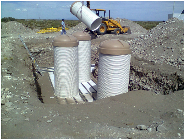
Fig. 3: Deployment of the first twin at Kathy-Turner when installing the service-tubes right before burying the modules.
