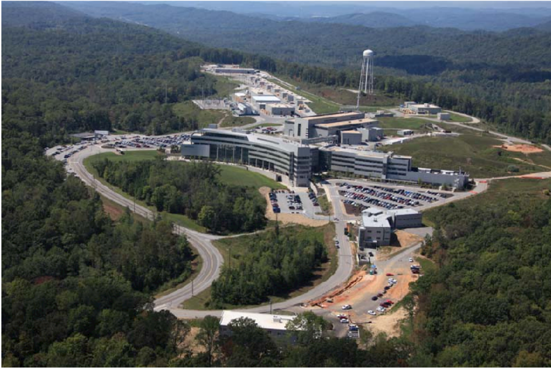
Figure 4.2: A photograph of the completed SNS facility.
