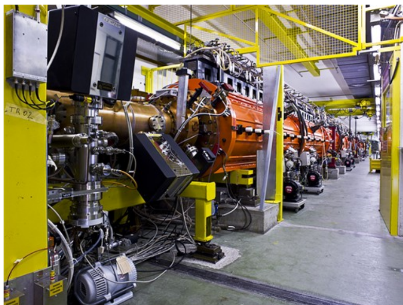
Fig. 4: RFQ2 and Linac 2 tanks
