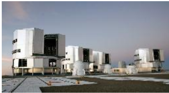
Figure 3: The Very Large Telescope operated in Chile by the European Solar Observatory. The light collected by four 8 m diameter mirrors (up to 130 m apart) can be recombined on the same detector.
