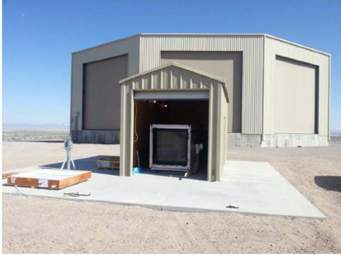
Figure 4.19: A photograph showing the shed housing EUSO-TA at the Telescope Array Black Rock Mesa site. The Telescope Array fluorescence detector can be seen in the background. The EUSO-TA optics (two Fresnel lens of  $1 \text{ m}^2$ ) have already been installed and can be seen inside the shed.
