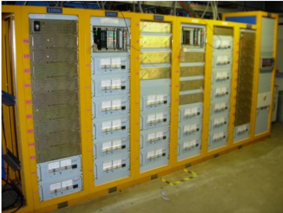
Figure 4.100. M4 beamline vacuum station located at AP30 service building will be reused.
