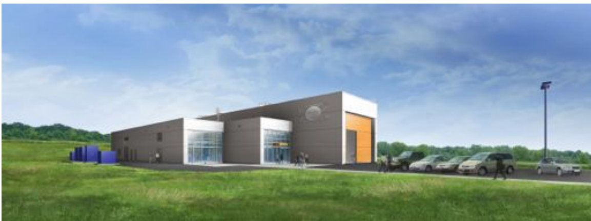
Figure 5.1. Entry View of the Mu2e facility, looking northwest.
