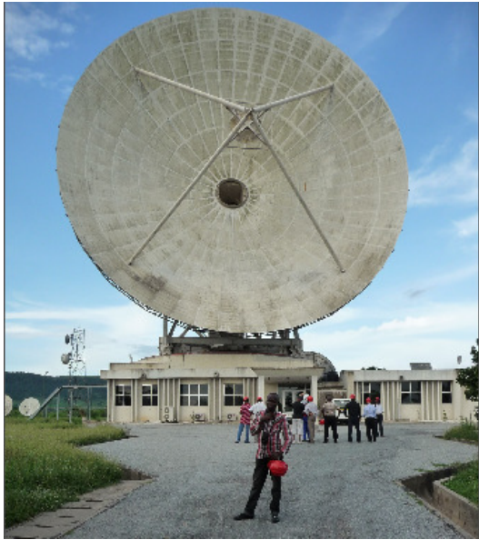
Figure 1. Left: The Kuntunse 32m disuse telecommunication antenna currently being converted to radio astronomy facility. Standing in front of the telescope is the first author. Right: African Undersea Cables span the coasts of Africa and link the continent to the outside World and represents greater internet bandwidth availability and potential of data transport from the Ghana antenna site [11].
