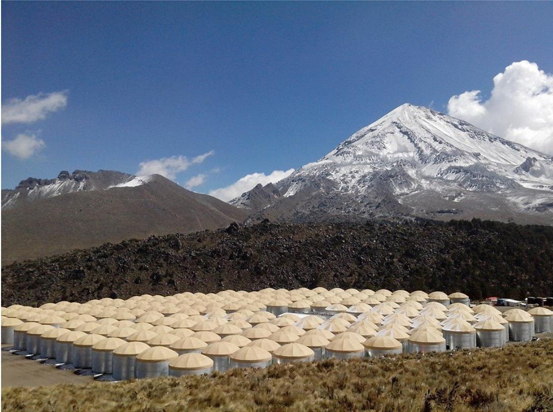
**Figure 2:** The High Altitude Water Cherenkov Observatory at its home near Pico de Orizaba in Mexico. The 300 WCDs are large and close-packed giving the instrument a footprint of 20,000 m<sup>2</sup>.
