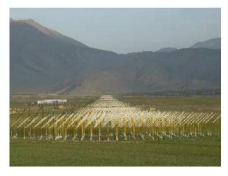
**Figure 1.** Photograph of the east-west baseline of the 21CMA, in which the building to the left is the control center.
