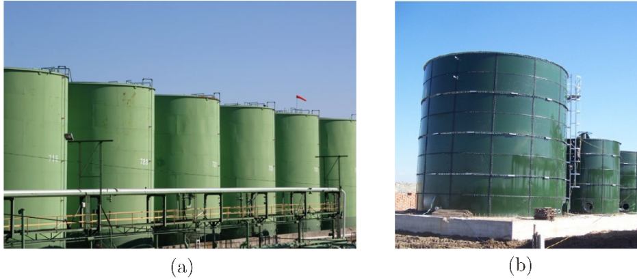
Figure 1: (a) Array of tanks in a petrochemical plant (image taken from www.joc.com , accessed on 19/01/2016); (b) cylindrical steel tanks, used to storage water, resting on a concrete foundation (image taken from www.alibaba.com , accessed on 19/01/2016).
