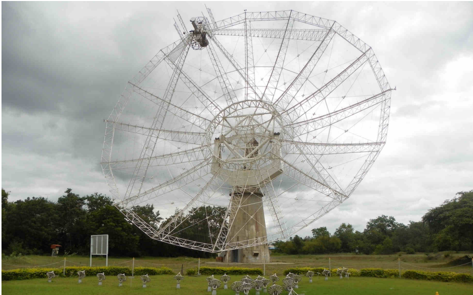
Figure 2.5. The Giant Metrewave Radio Telescope (GMRT) is composed of 30 antennas with a diameter of 45 m each. The largest separation between them is 25 km.
