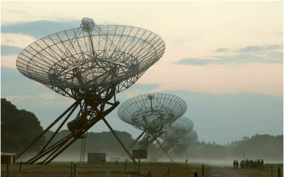
Figure 2.4. The Westerbork Synthesis Radio Telescope (WSRT) is composed of 14 antennas with a diameter of 25 m each. The largest separation between them is 2.7 km.
