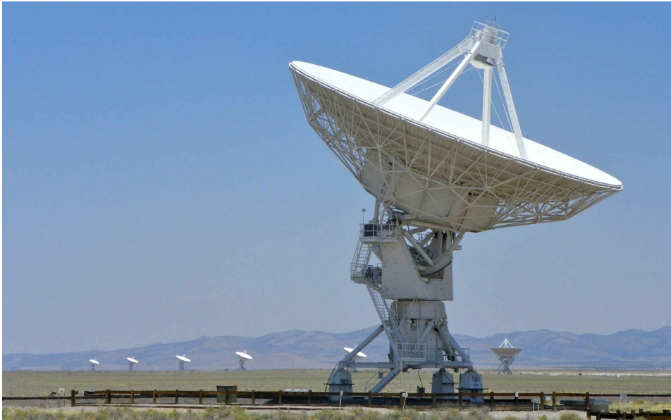
Figure 2.3. The Karl G. Jansky Very Large Array (VLA) is composed of 27 antennas with a diameter of 25 m each. The largest separation between them is 36.4 km.
