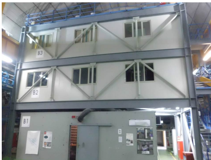
Figure 29: A picture of the existing OPERA CS facility in hall B.
