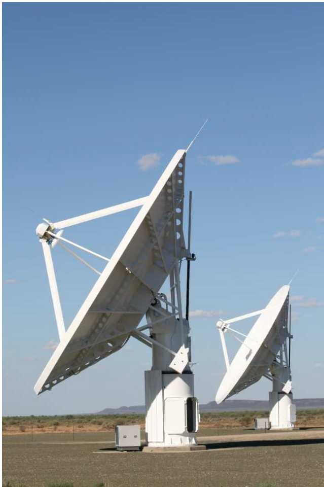
Figure 3. Two of the KAT-7 dishes viewed side-on. Note the lightning rods at the apex and near the focus, the backing structure of steel beams with circular holes, the small counterweight on the right and the sun shield on the left hand side of the pedestal.
