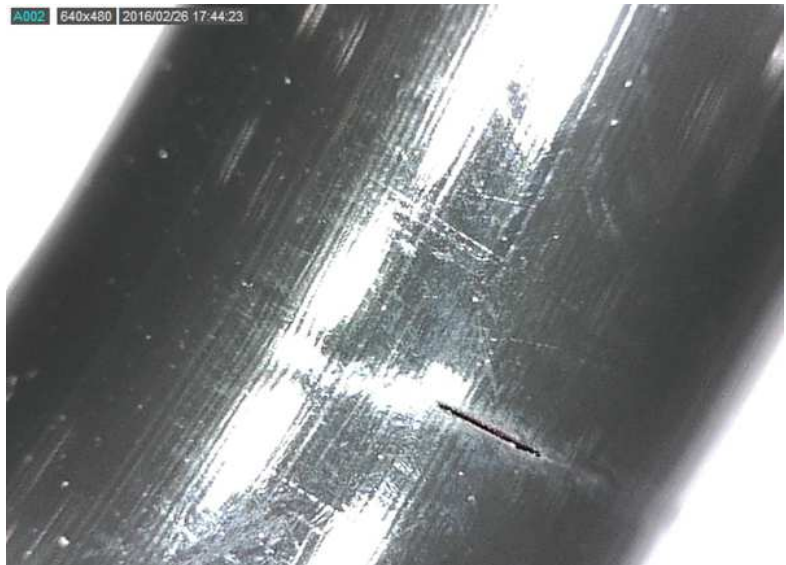
Figure 8. A rupture in an internal cooling line (shown here) led to a damaging glycol leak during the 2016A run. The outer diameter of the hose is 8mm. The crack was along the outer curve of a bend, and pointed almost straight down when mounted and with the telescope at zenith.
