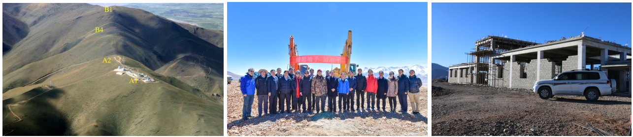
FIG. 4: From left to right: aerial view of the region around Ali Astronomical Observatory (5100m at A1), picture for laying the foundation for AliCPT at B1 point (5250 m), the current infrastructure for AliCPT.
