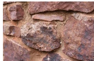
Figure 5. The red stone scattering surface.
