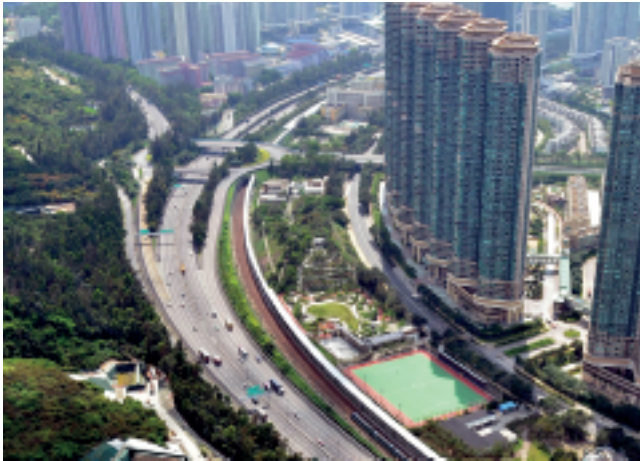
Figure 1. Cost and completion time information for 25 completed Hong Kong road projects was retrieved and analysed
