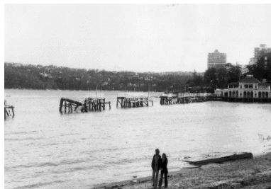
1974 - Damaged boardwalk, Manly Cove 1
