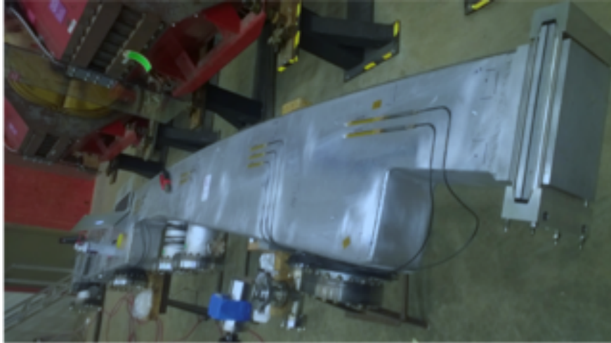
Figure 6: Vacuum chambers with monitoring NMR probes installed in the grooves.
