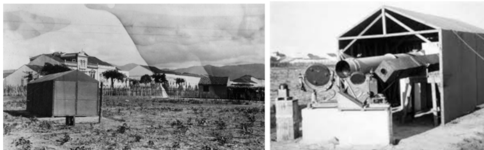
FIG. 31: Left: The British tent closed. The Saboya house is in the background. Compare with the previous photograph. Right: The British tent opened with the two telescopes used by Crommelin and Davidson, the 4 inch telescope on the right and the 13 inch astrographic telescope on the left, together with the respective coelostats. The telescopes are pointing eastward as the eclipse was to be at 9:00am. Courtesy of the Royal Greenwich Observatory.
