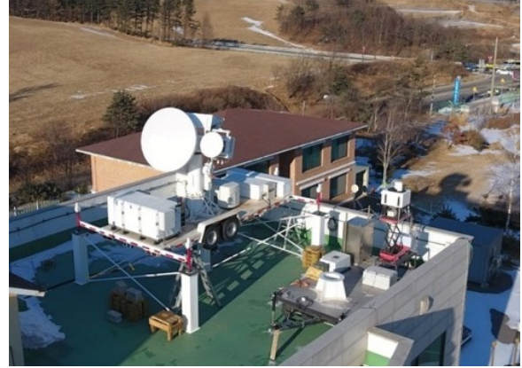
Fig. 1: The NASA D3R deployed at rooftop of DaeGwallyeong Regional Weather Office (DGW) in the daegwallyeong-myeon province of South Korea.
