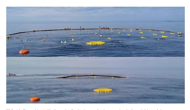
FIG. 10. Two video stills from the final minute of valve opening before sinking of the 3D-T mooring array.
