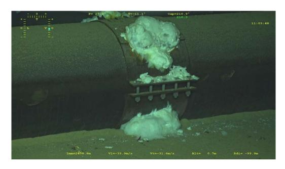
FIG. 14. Detail of cable attachment saddle with heavily deteriorating zinc-aluminum-alloy anode.
