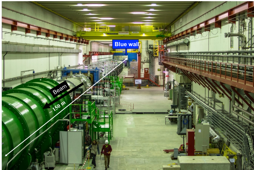
Figure 4. View of the ECN3 hall hosting the NA62 experiment.
