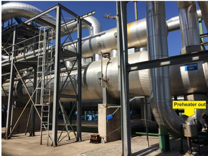
Figure 7. Sampling points in the surface equipment system of the GGF (Photo credit: Beştepeler company)
