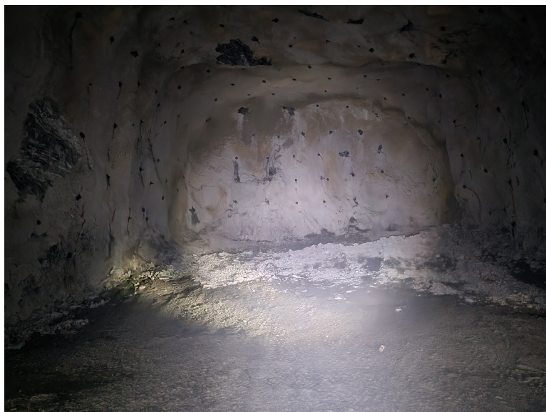
Figure 22. Completed Cyclotron Room excavation.
