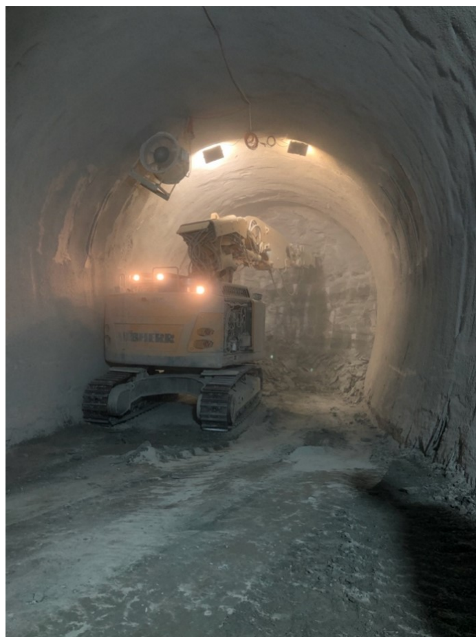
Fig. 21. Rockbreaker used for cavern excavation at HL-LHC Point 1
