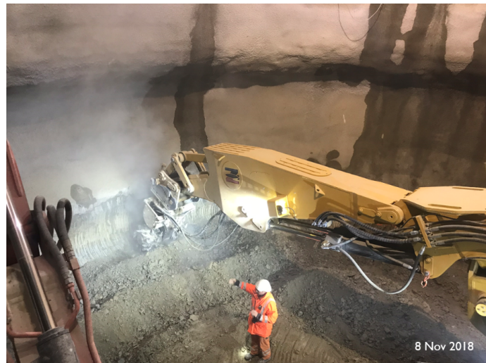
Fig. 20. Excavator with hydraulic cutting heads being used at HL-LHC Point 1
