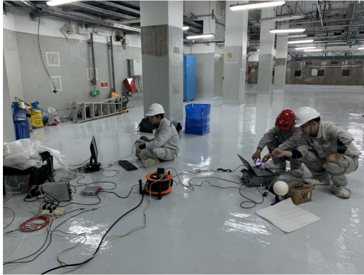
Figure 3: The interior of the basement where TAO will be located. Cable trays along the wall and gas and water pipes on the ceiling can be seen.
