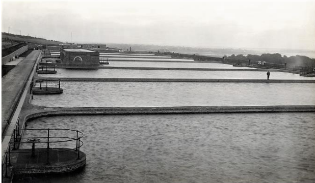
Figure 1 - Large-scale slow filtering. Portsmouth, 1927
