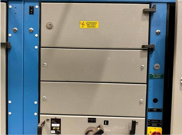
Figure 38: Picture of the spare feeders available in the existing EBD1/4X.
