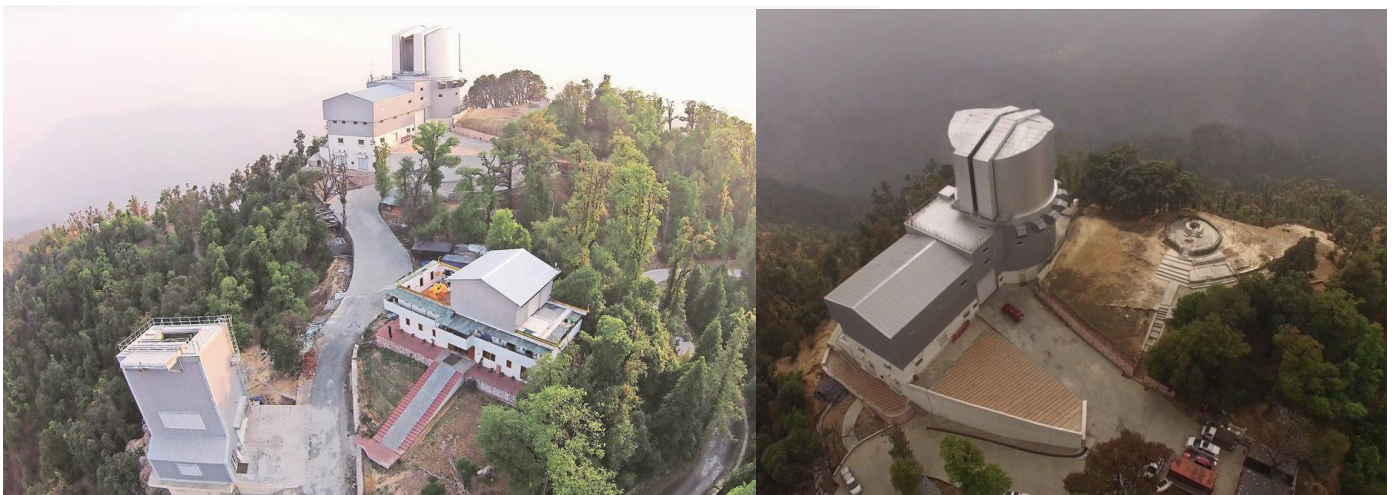
Figure 1. Devasthal Observatory hosting the (a) 1.3 m DFOT building with the sliding roof (bottom right) and rectangular building of the 4 m ILMT (bottom left), and (b) 3.6 m DOT near the adjacent Devasthal temple.
