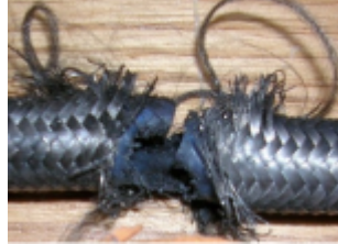
Figure 2: The power cable of ISS, damaged by the collision of debris [31].
