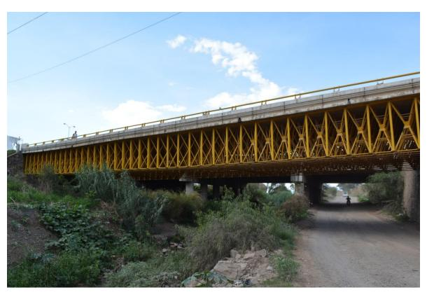
Figure 1 Tridilosa Bridge
