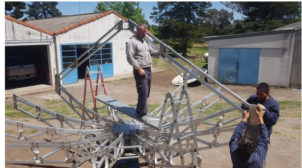
Fig. 12. First parabolic dish under construction.
