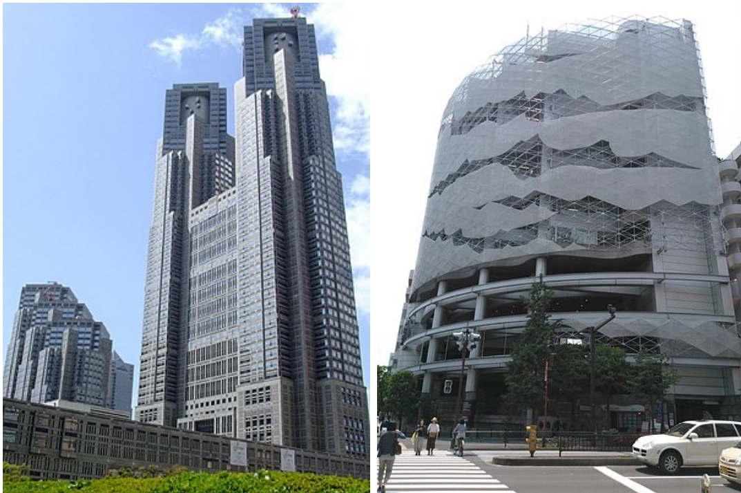
(a) Metropolitan Government Building.
