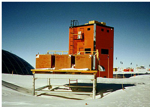
Figure 1: Photo of the three detector tubes in the initial installation of the NM-64 neutron monitors at the South Pole. The neutron monitors are on an elevated platform in insulated, heated boxes. Also shown in the background are the Skylab building (housing the monitor electronics, among others) and part of the iconic Dome (credit: L. Shulman/Bartol).
