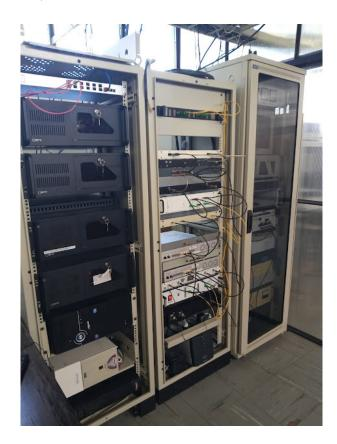
Fig. 22. Digital back-end based on ROACH boards developed by CASPER collaboration and storage in the control room of IAR's radio telescopes.
