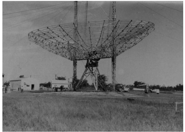
Fig. 5. Mounting the radio telescope disk on its pedestal. 1965.
