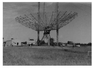
Fig. 5. Mounting the radio telescope disk on its pedestal. 1965.
