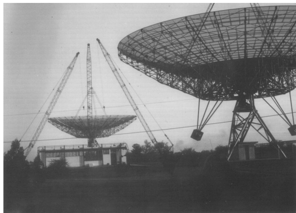
Fig. 10. Assembly of the second IAR radio telescope, 1973.
