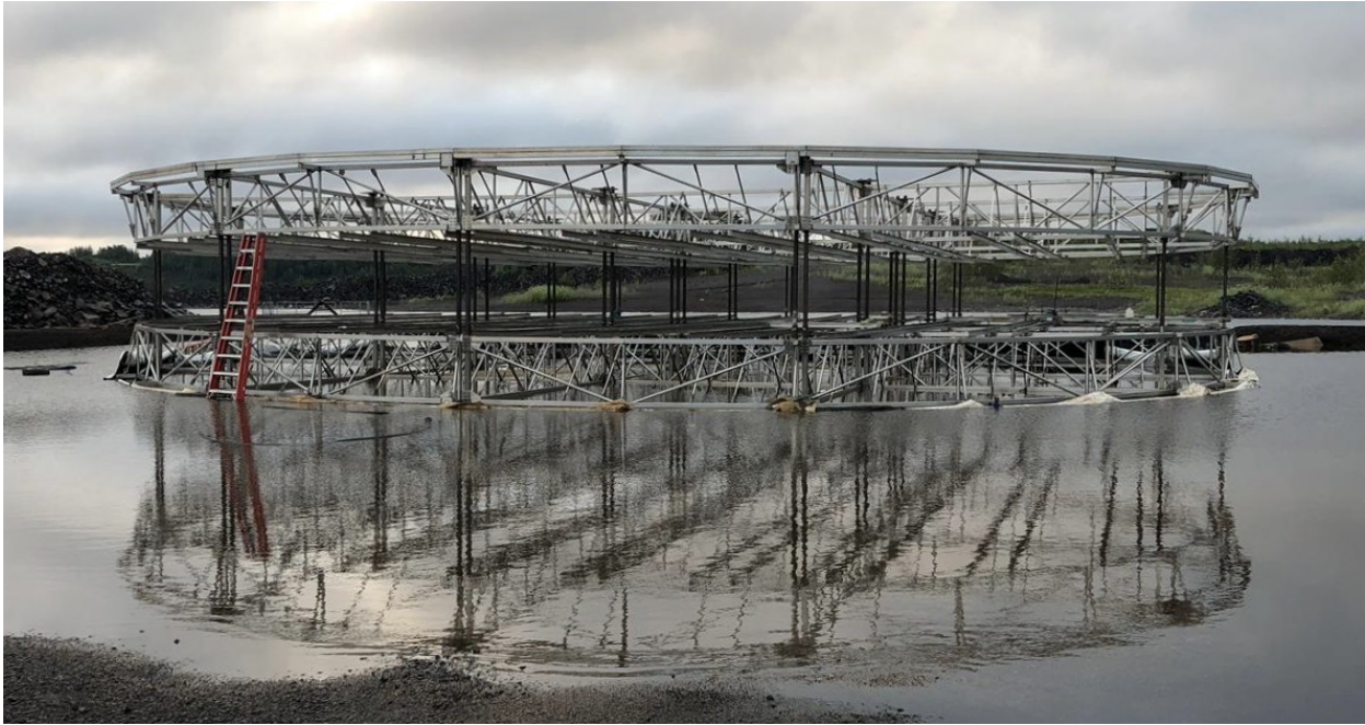
Figure 5: Completed frame. The pillars supporting the top cap are clearly visible.
