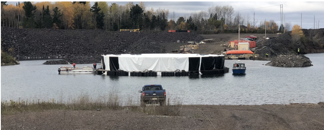
Figure 13: The exterior of the detector after completion. The liner can be seen supporting the detector and the floating dock forms a perimeter around the detector. Two boats tow and steer the detector during deployment. The scale of the detector is visible.
